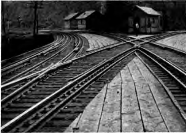
P. & M. Rail Anti-Creepers Anchoring Approach to Pittsburgh & Lake Erie Railroad Bridge, McKeesport, Pa.
